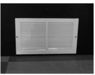
When the flow is limited or inaccessible between rooms downstairs (if there are walls or partitions), then install a grille 8" x 10" (or other grill configuration, having total area of not less than 80 sq. in.) in the bottom of the door or wall to avoid having stagnant air in those areas. Otherwise interior doors must remain open. This insures that all the air drawn into the Humidex comes from all areas of the basement.
