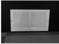
When the flow is limited or inaccessible between rooms downstairs (if there are walls or partitions), then install a grille 10" x 14" (or other grill configuration, having total area of not less than 100 sq. in.) in the bottom of the door or wall to avoid having stagnant air in those areas. Otherwise interior doors must remain open. This insures that all the air drawn into the Humidex comes from all areas of the basement.
